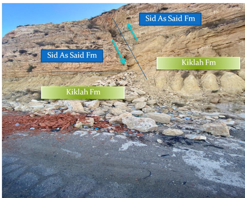
Figure (4): Picture of Fault, Showing the Threat Posed this Fault Instability on Road Users.
